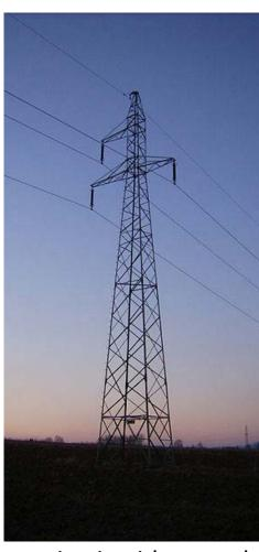
single 3-phase circuit with ground wire
